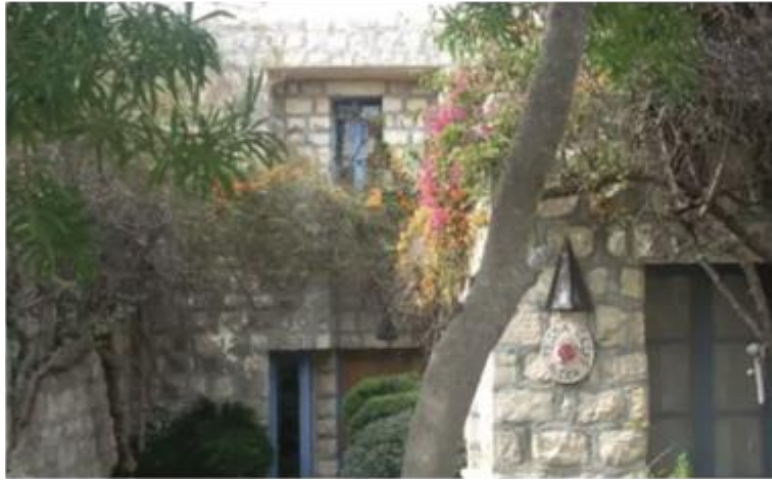
Renovated House, Recent visit
