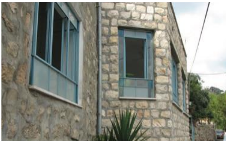
Renovated House, Recent visit
