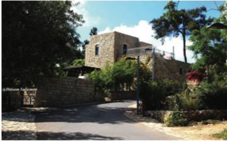
Renovated House, Recent visit
