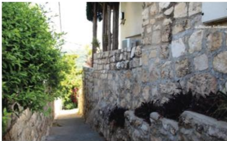
Renovated House, Recent visit
