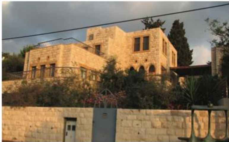
Renovated House, Recent visit
