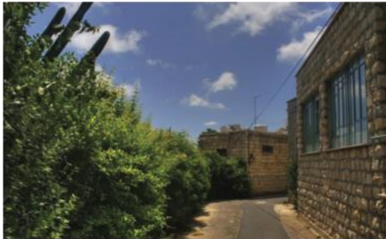
Renovated House, Recent visit
