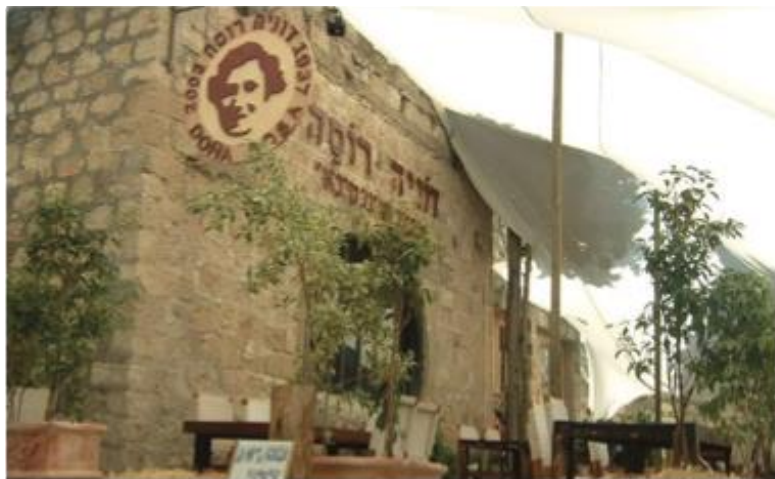
Renovated House, Recent visit
