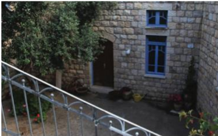
Renovated House, Recent visit
