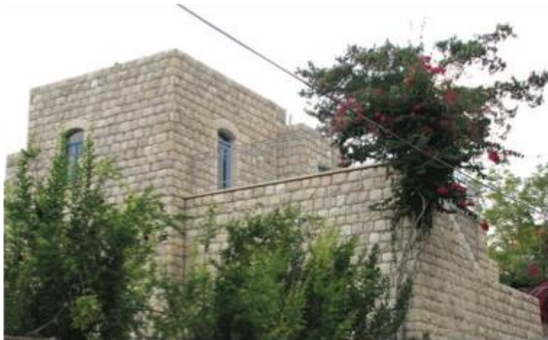
Renovated House, Recent visit
