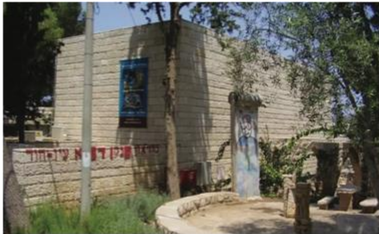
Renovated House, Recent visit
