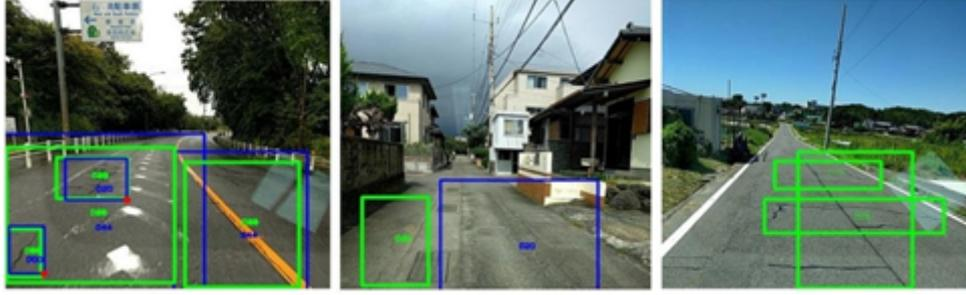
**Figure 2.2:** Classification of predicted crack examples: True Positive-(a), False Positive-(b), False Negative-(c) obtained from YOLO v2 in [44]
